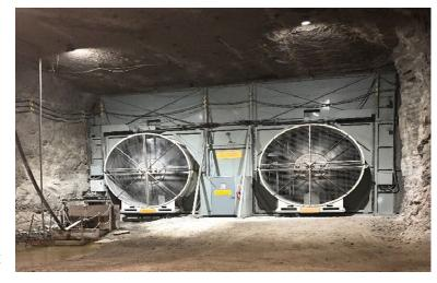
stalled, clearing the shot took six to eight hours, but now only one hour. Repositioning is accomplished remotely from the surface, in four minutes, using motors and cameras to verify position, thereby removing any potential safety hazard to miners. Rotating the fans also allows the company to manage potential ice buildup in the ventilation shaft or decline road into the mine.
