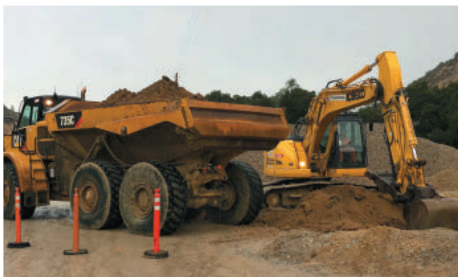
Construction of new pond up gradient of existing pond.
